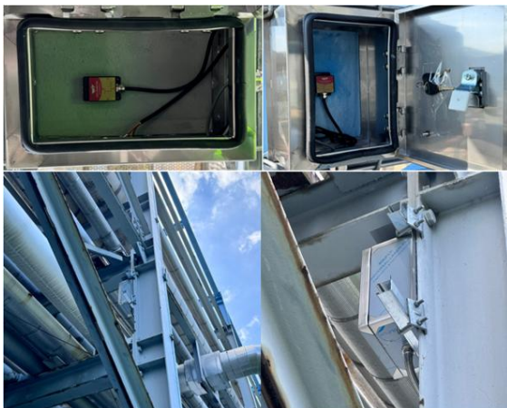
Figure 5: Installation Status of Pipe-rack Sensors
