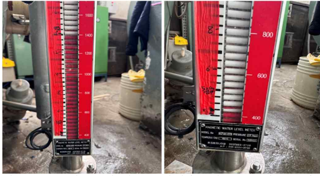
Figure 3. Magnetic water level meter. The left panel represents the state after washing water supply, while the right panel represents the state before dyeing wastewater effluent discharge.
